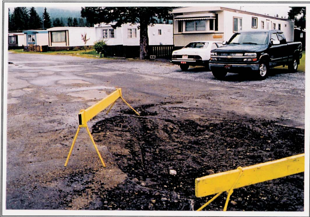
Plate 1 View southeast of mobile homes in Restwell Trailer Park. Large backhoe test in foreground.
