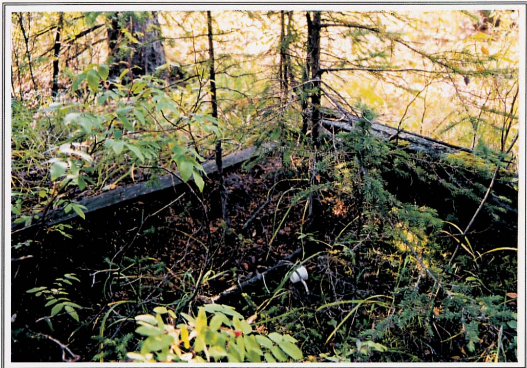
Plate 9 View southwest of Feature 2. Wooden foundation of recent materials abandoned about 1988.
