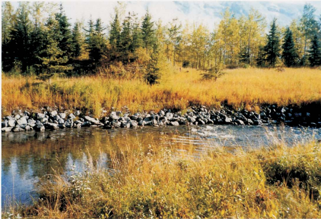
Photo V-5 Riprap Bank Armoring along Right Downstream Bank, Approximately 2 km Upstream of the Policeman Creek – Bow River Confluence (not part of Restwell property)
